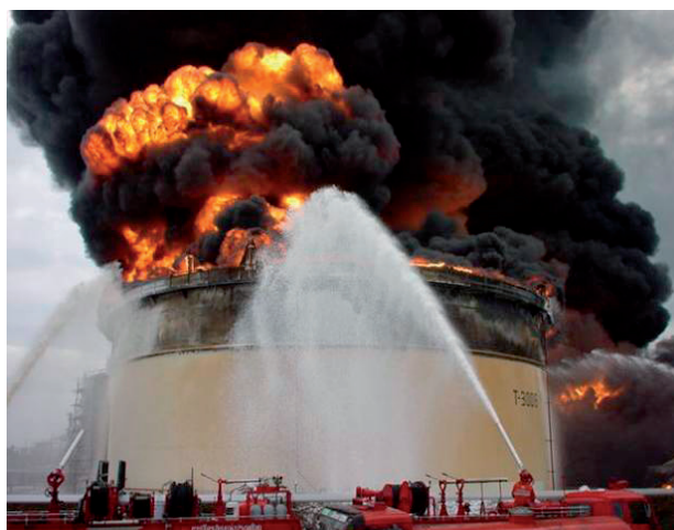
Fot. 9. Wyrzut ropy naftowej. [24] Pict. 9. BOILOVER of crude oil. [24]
